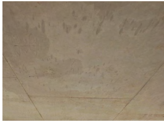
Rippling effect on concrete.
