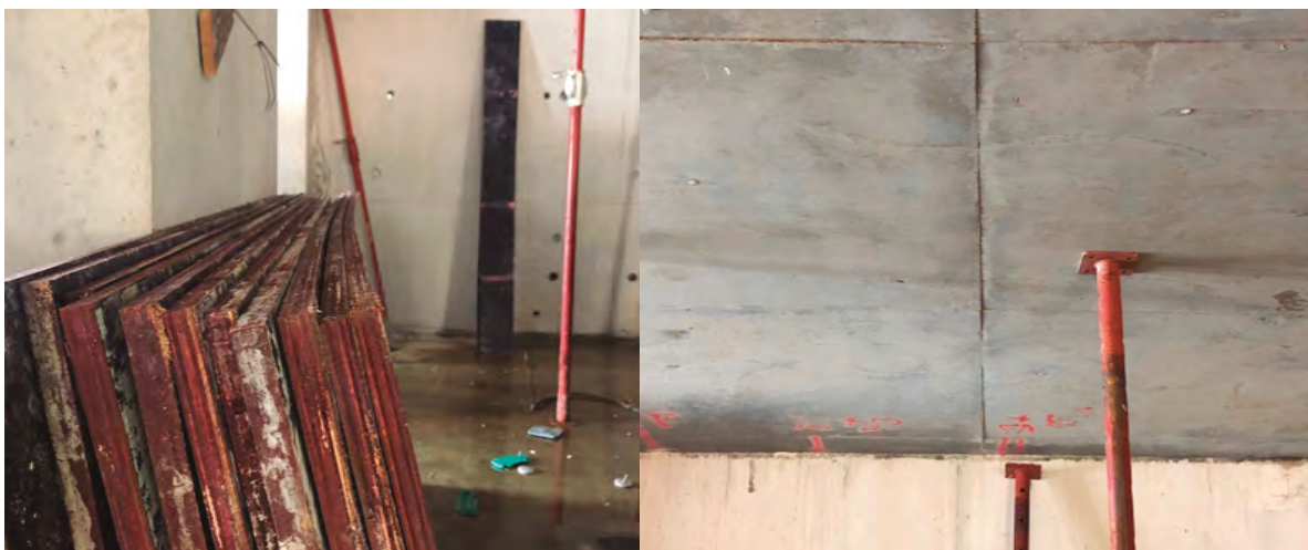
Incorrect shoring between panels.
