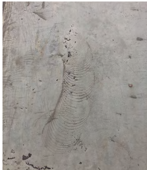
Mark left in the concrete by the vibrator.
